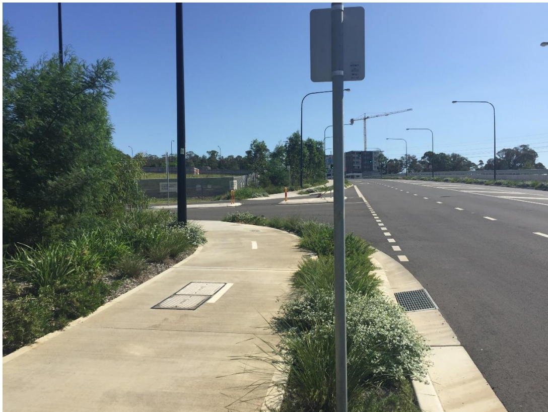
Photo 2 – Cudgegong Road / Conferta Avenue Intersection
